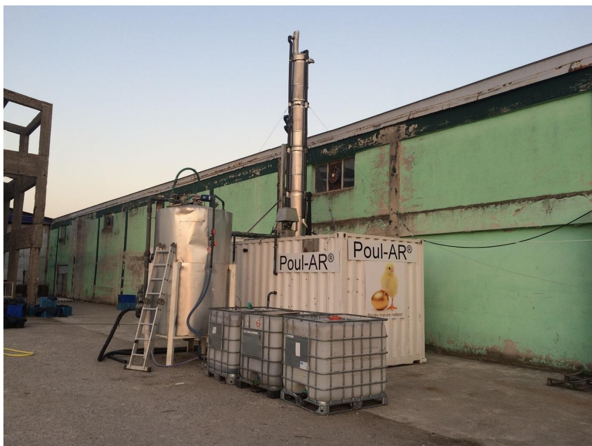
Figure 1: Poul-AR pilot installation in Karacabey (Bursa, Turkey) at Burdan Egg
